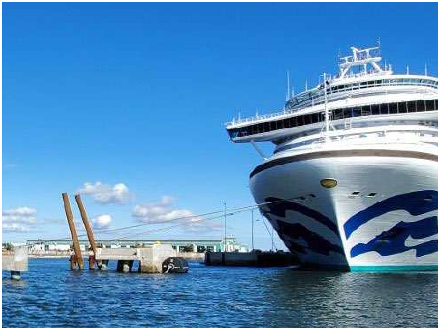
PORT CHARLOTTETOWN CANADA CRUISE TERMINAL
